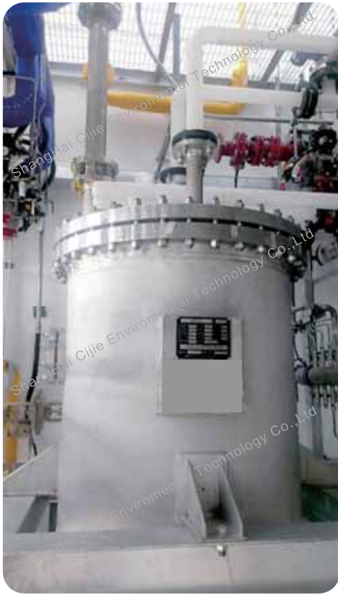
Catalyst recovery – stainless steel lined PTFE
